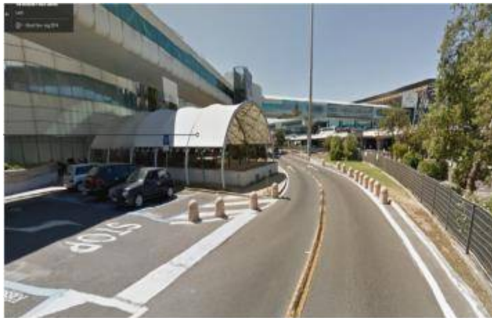
BEFORE WORKS PICTURE
