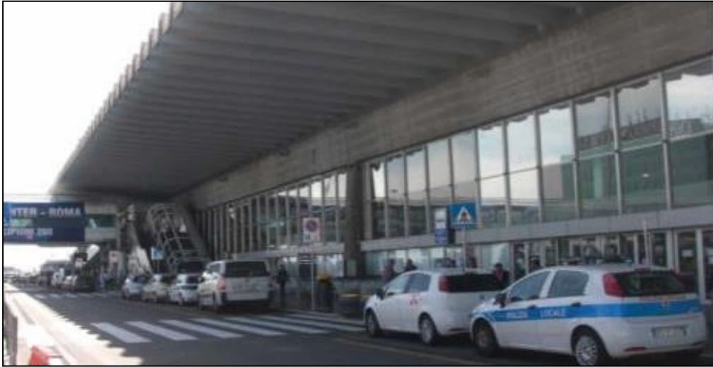
2015: outside T3 before starting facade upgrade
