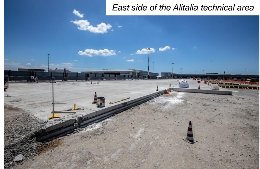
East side of the Alitalia technical area
