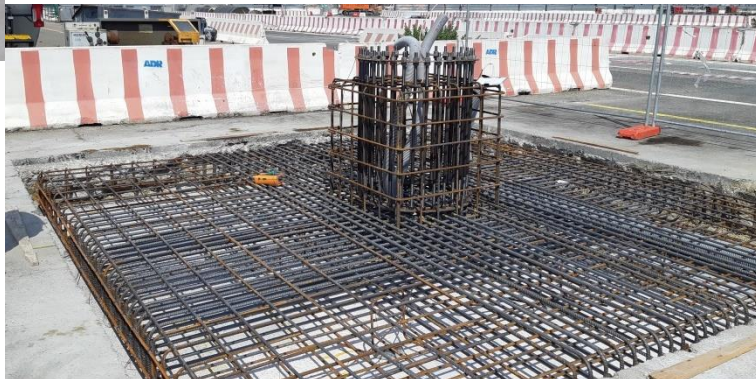
Construction of a new base for the light tower
