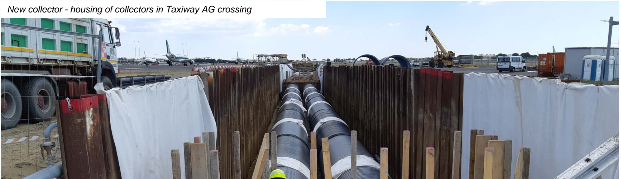
Building of oil separator tank in reinforced concrete West RWY 16R/34L
