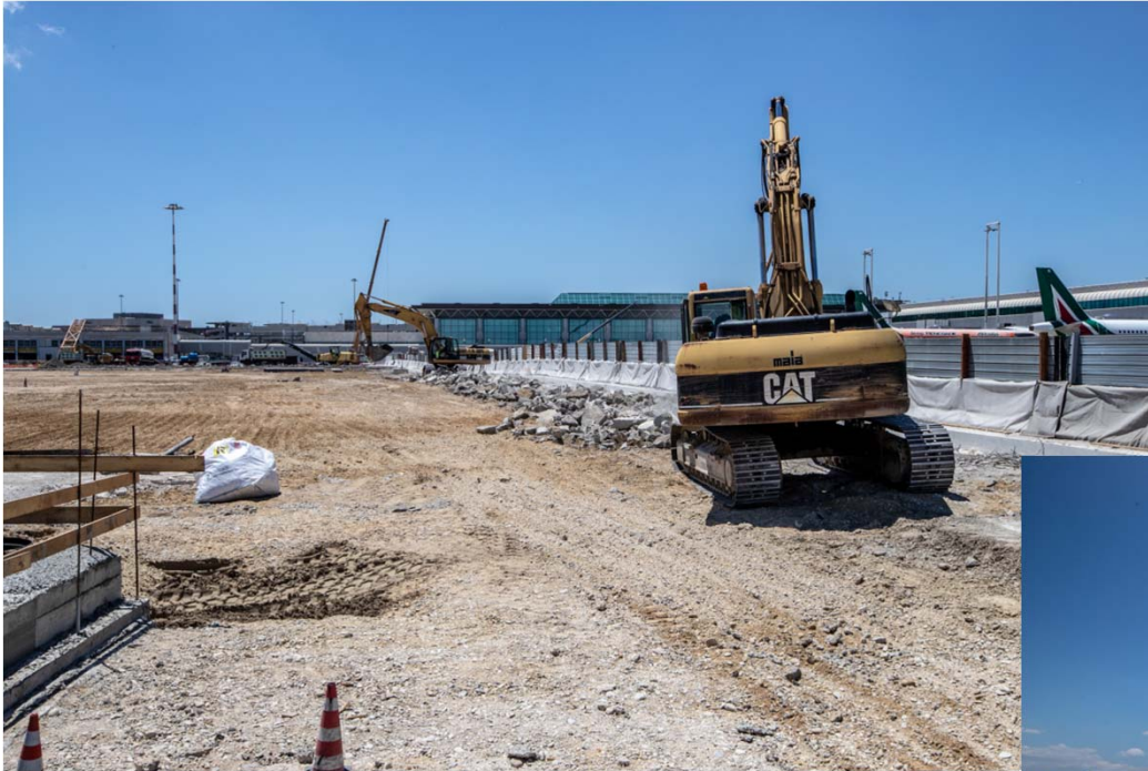
West front, quadrant 400 side
