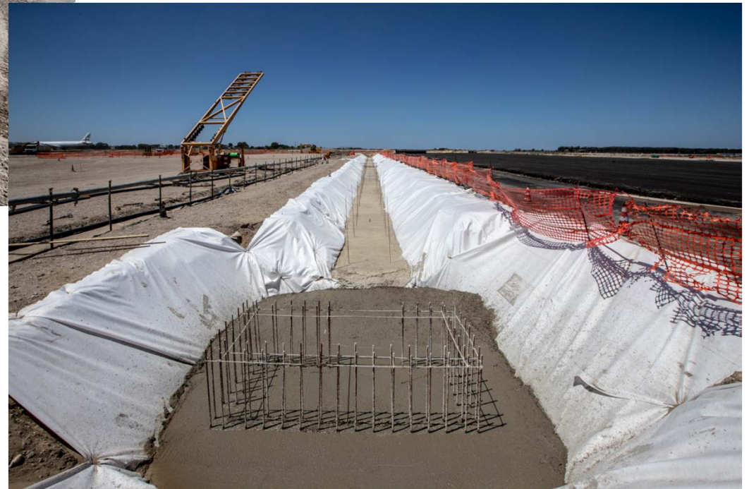
West Area phase 2 - Execution of water works
