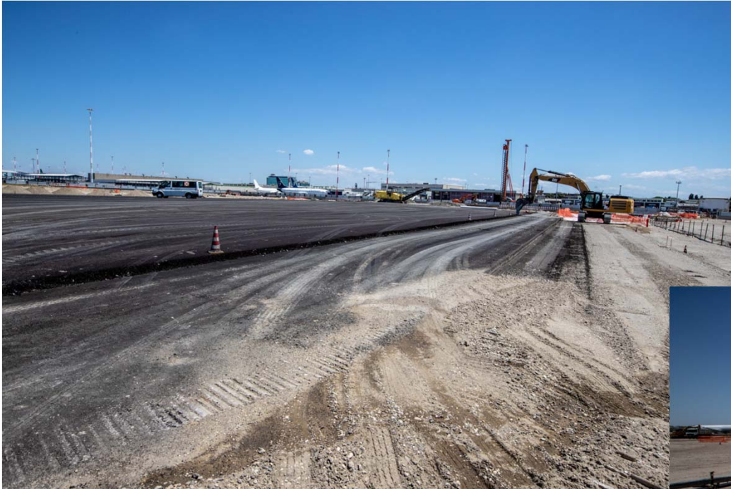
West Area phase 2 - Laying of flexible paving
